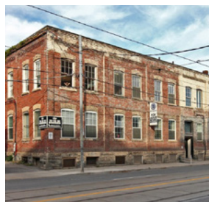
dufferin street, toronto 45,000 sf office building june 2016
