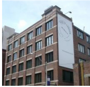
richmond street west, toronto 40,000 sf office building may 2004
