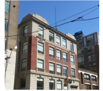
adelaide street west, toronto 40,000 sf office building may 2004
