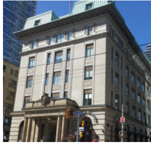
king street west, toronto 76,000 sf office building may 2013
