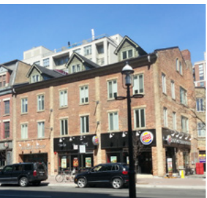
front street east, toronto 34,000 sf office building april 2007
