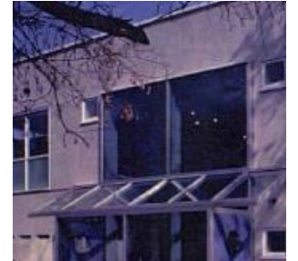
bishop street, toronto 5,000 sf office building september 2003
