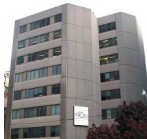
st.clair avenue west, toronto 34,500 sf office building february 2004
