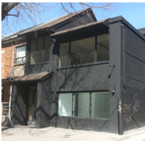
richmond street west, toronto assembly - 2,500 sf april 2012
