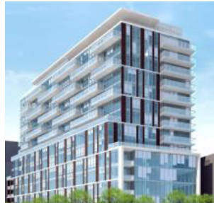
king street east, toronto 18,000 sf development site january 2008
