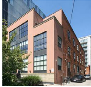
wellington street west, toronto 60,000 sf future development july 2020
