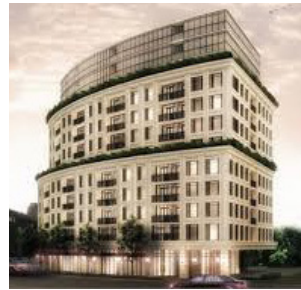
davenport road, toronto 12,000 sf development site july 2012
