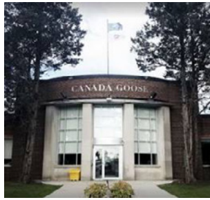
bowie avenue, toronto 7 acre mixed use development site march 2022
